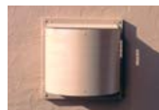
AstroCap™ horizontal venting system (279mm X 279mm X 165mm)
